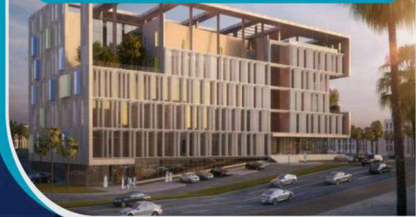
ADVANCED MANUFACTURING BUILDING, KSA
